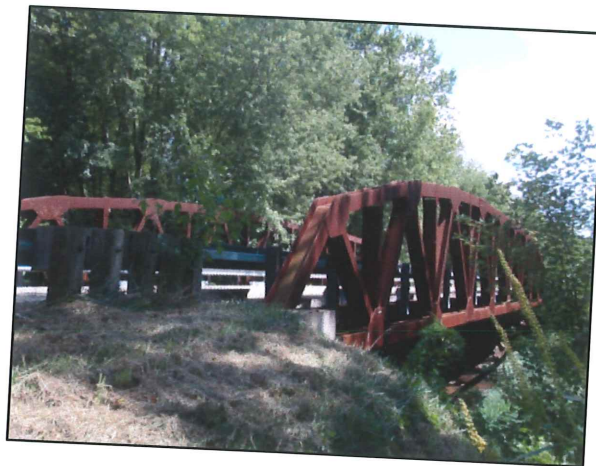
Figure 1 – SFN 4930975 – Elevation looking northeast
