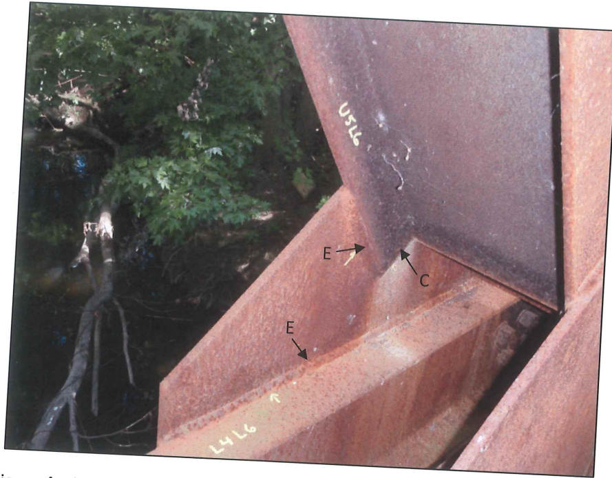
Figure 4 – Longitudinal and transverse fillet welds connecting truss members to the gusset plates.
