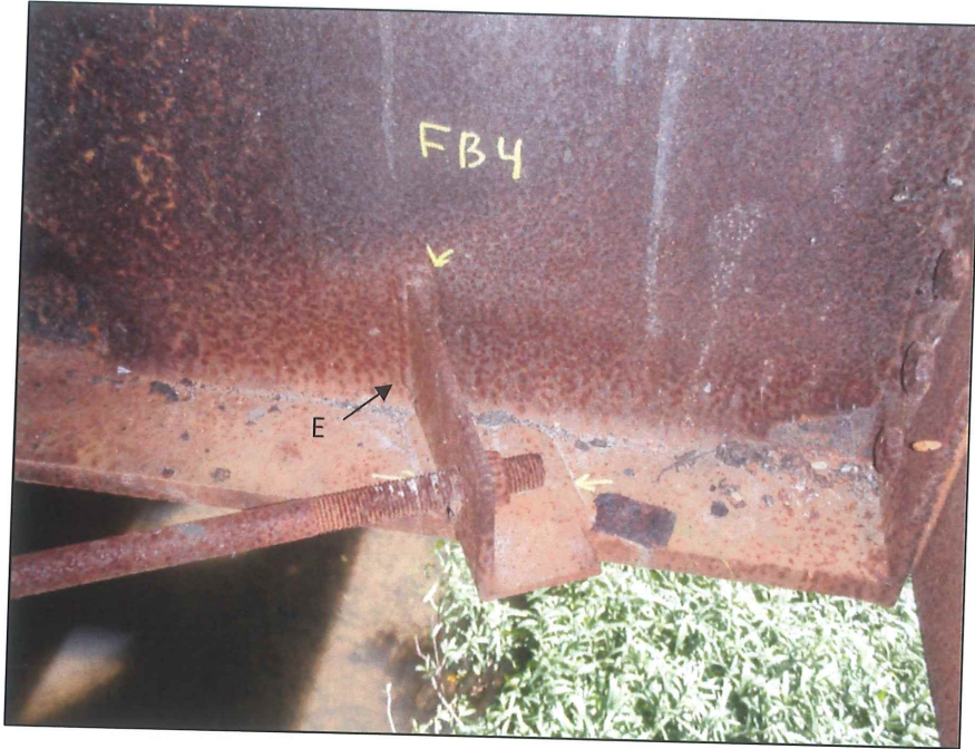
Figure 6 – Lower Lateral Bracing connection to Floorbeam 4. Note: Fillet welds on the web and bottom flange of the floorbeam.
