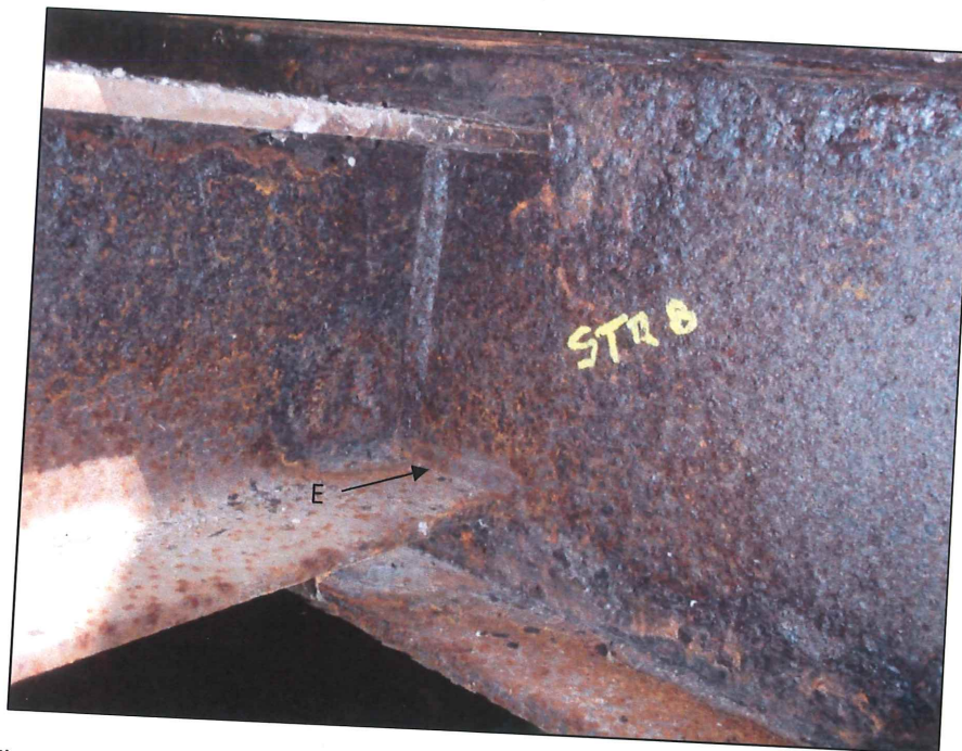
Figure 5 – Guardrail post connection to Stringer 8. Note: Welds on the web of the stringer.
